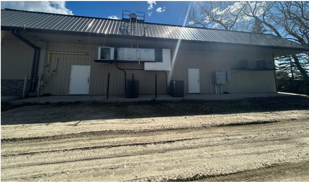
WEST SIDE OF BUILDING
