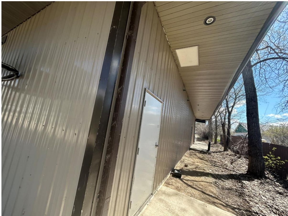
SOUTH SIDE OF BUILDING
