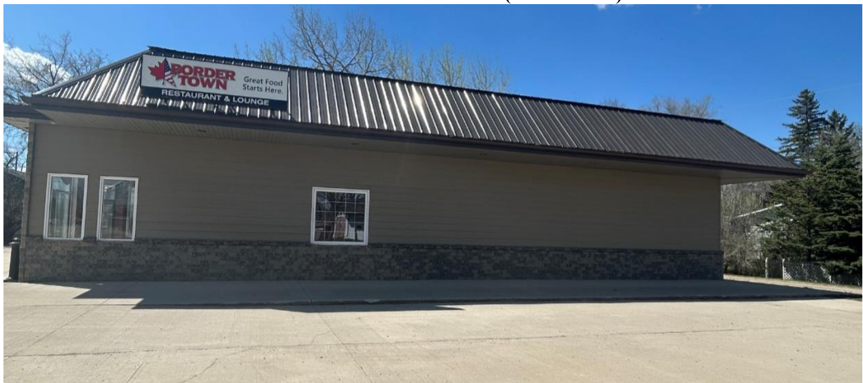
NORTH SIDE OF THE BUILDING & PARKING LOT
