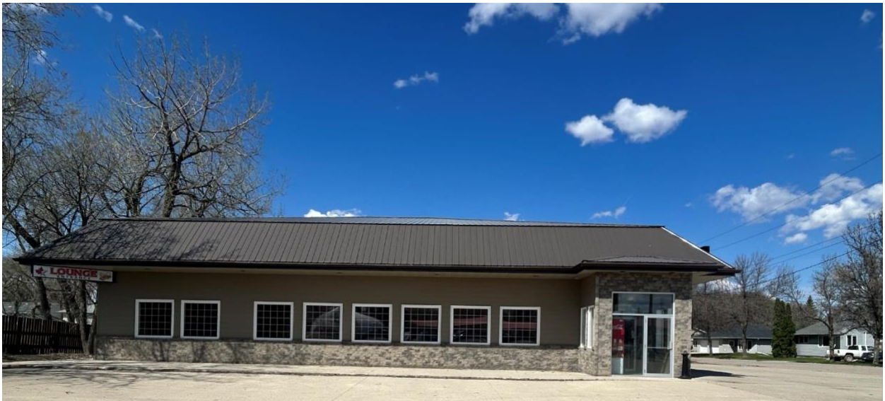
FRONT OF THE BUILDING (EAST SIDE)
